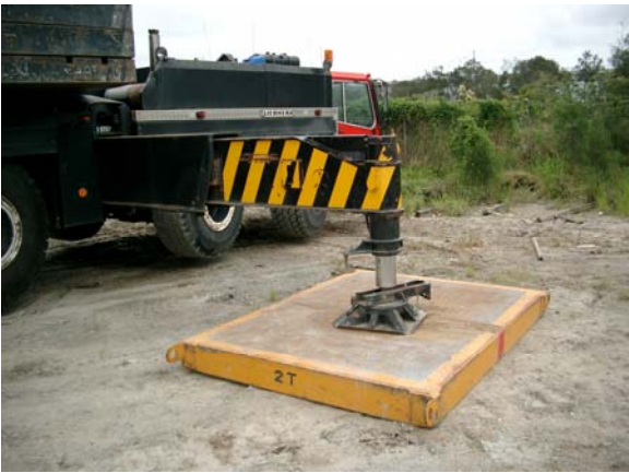
Figure 4 - Crane outrigger foot on bog mat
