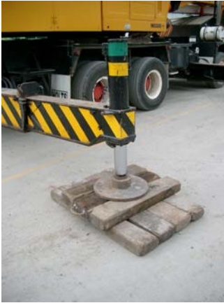
Figure 3 - Crane outrigger foot on timbers
